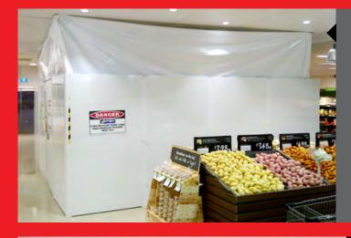
ZipWall<sup>®</sup> can be used in conjunction with lower height hoarding systems such as Hoardfast<sup>™</sup> in retail environments or other public spaces to give a floor to ceiling dust seal with the solid security and privacy hoarding up to eye-level.
