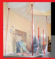
Use in conjunction with portable self-contained air filtration machines. These units can be used in enclosed areas as stand alone air scrubbers or built into the ZipWall<sup>®</sup> barrier to create negative air pressure.
