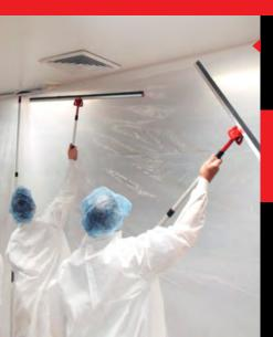
Connect 1.5m Tight-Seal rails to ZipWall<sup>®</sup> poles to create a tighter seal against the ceiling.
