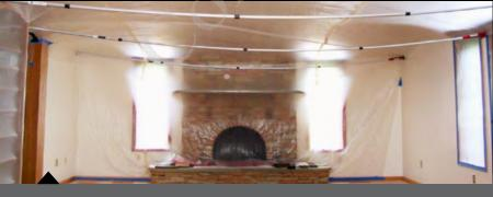
ZipWall<sup>®</sup> is so versatile it can be used for a range of random uses as broad as your imagination like this project above where the ceiling was protected from concentrated sanding dust by stringing the poles horizontally wall to wall!
